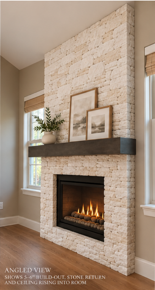
TOP DETAIL Stone scribed to sloped ceiling (ceiling rises into room)
